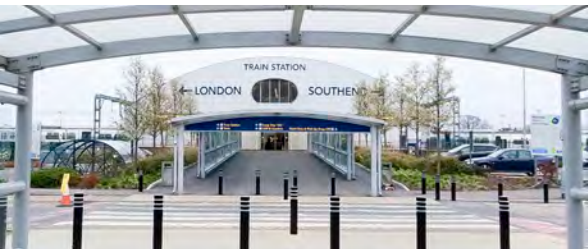
Figure 22: Train station identification at London Southend airport
